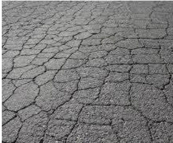
Figure 2.12 Fatigue 'alligator' cracking in asphalt pavement [126].
