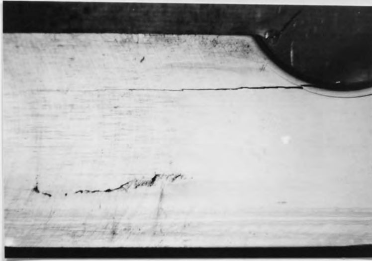
Figure 78: Longitudinal cracking in un-side-grooved 8090-T6 (L-S) specimens.
