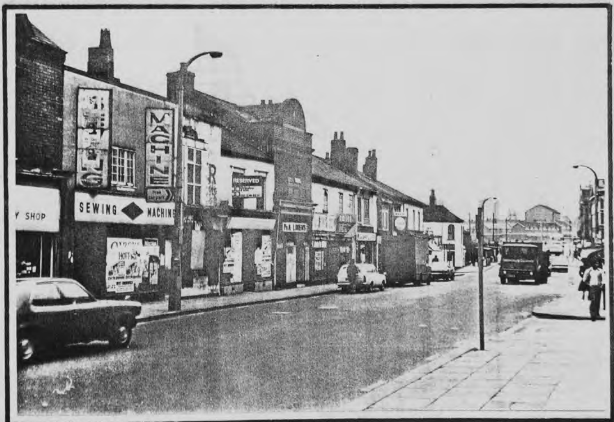
West Smethwick High Street: an example of inner urban decay due to demolition and depopulation of surrounding terraced streets. 80% of shops abandoned.
