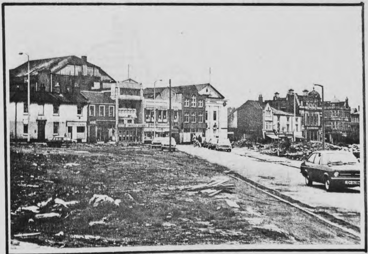
Smethwick; a commercial street, including cinema, bordering a derelict and demolished industrial site.
