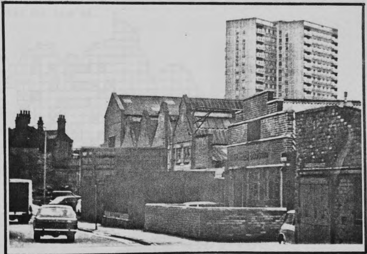
Modern Council tower-blocks overlook inner-city industrial buildings in Smethwick.
