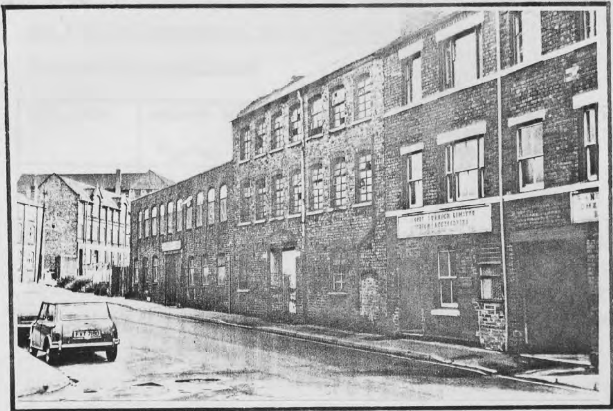
Densely-packed, Victorian inner-city industrial buildings in Walsall. Buildings frequently obsolete and in decay.
