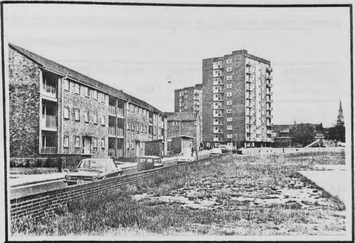
Council flats and surrounding recreational areas in Wolverhampton.
