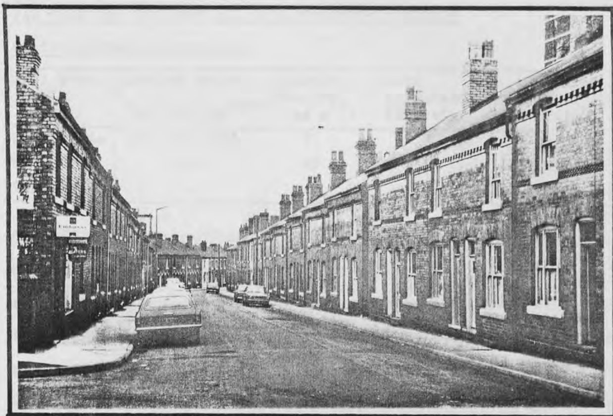
Typical inner-city Victorian working class terraced housing in Pleck, Walsall. Houses are of the 'two up, two down' type, fronting directly onto pavements devoid of front gardens or trees.
