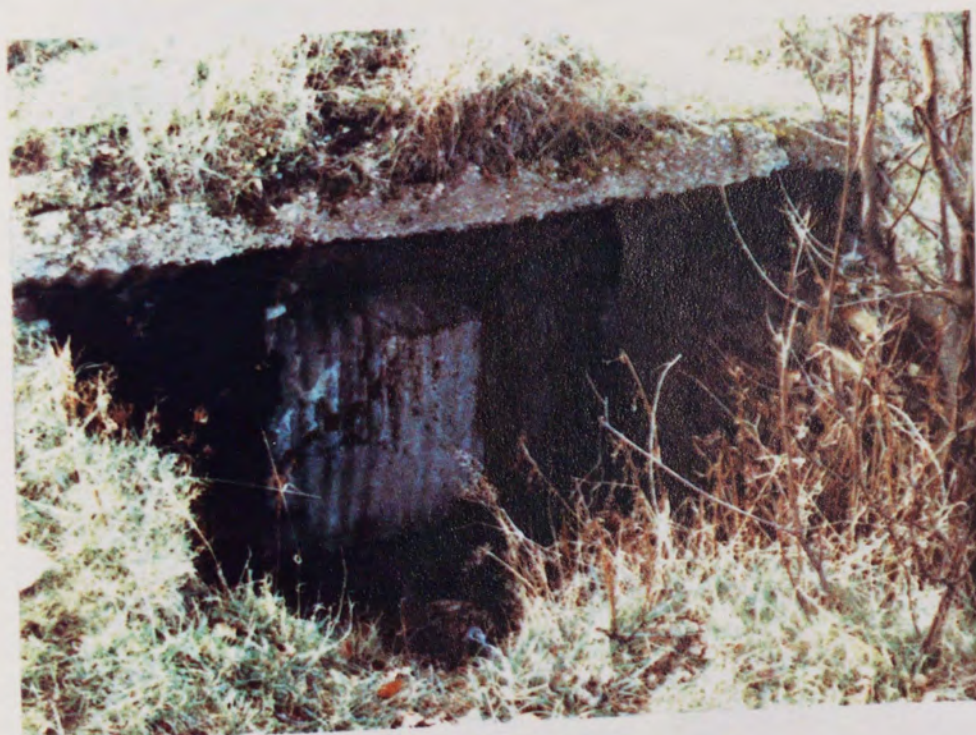
PLATE 5-3-2 Adit entrance. Nov, 1983.
