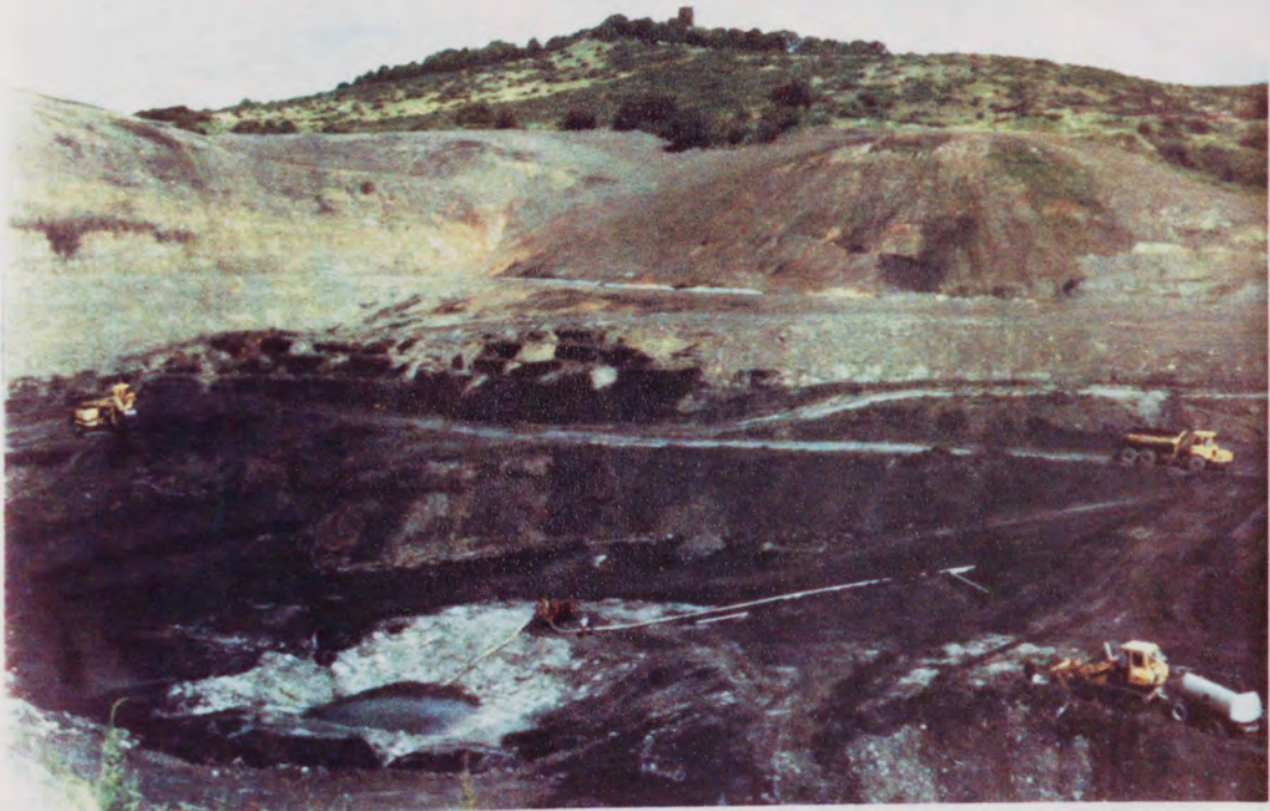
PLATE 5-3-8 Looking east over final excavation area - Heathen coals and Thick coal pickings exposed.
