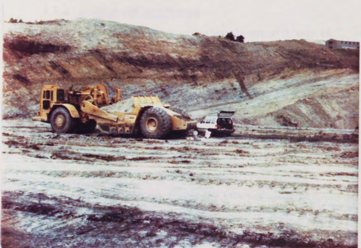
PLATE 5-3-12 Plate loading test. Aug. 1985.
