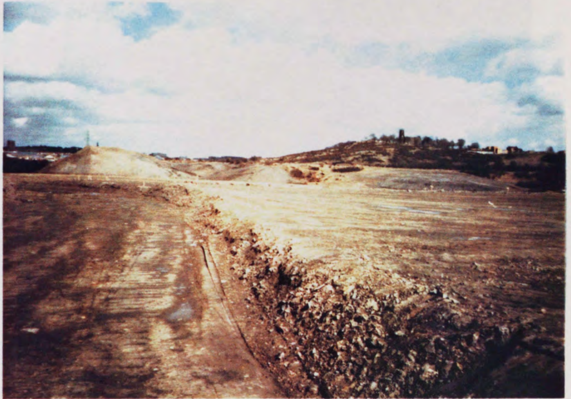
PLATE 5-3-3 Finished backfill area. March, 1986.
