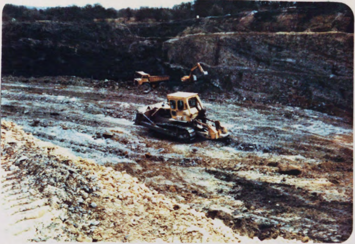
PLATE 5-3-5 Ripping the formation. April, 1983.
