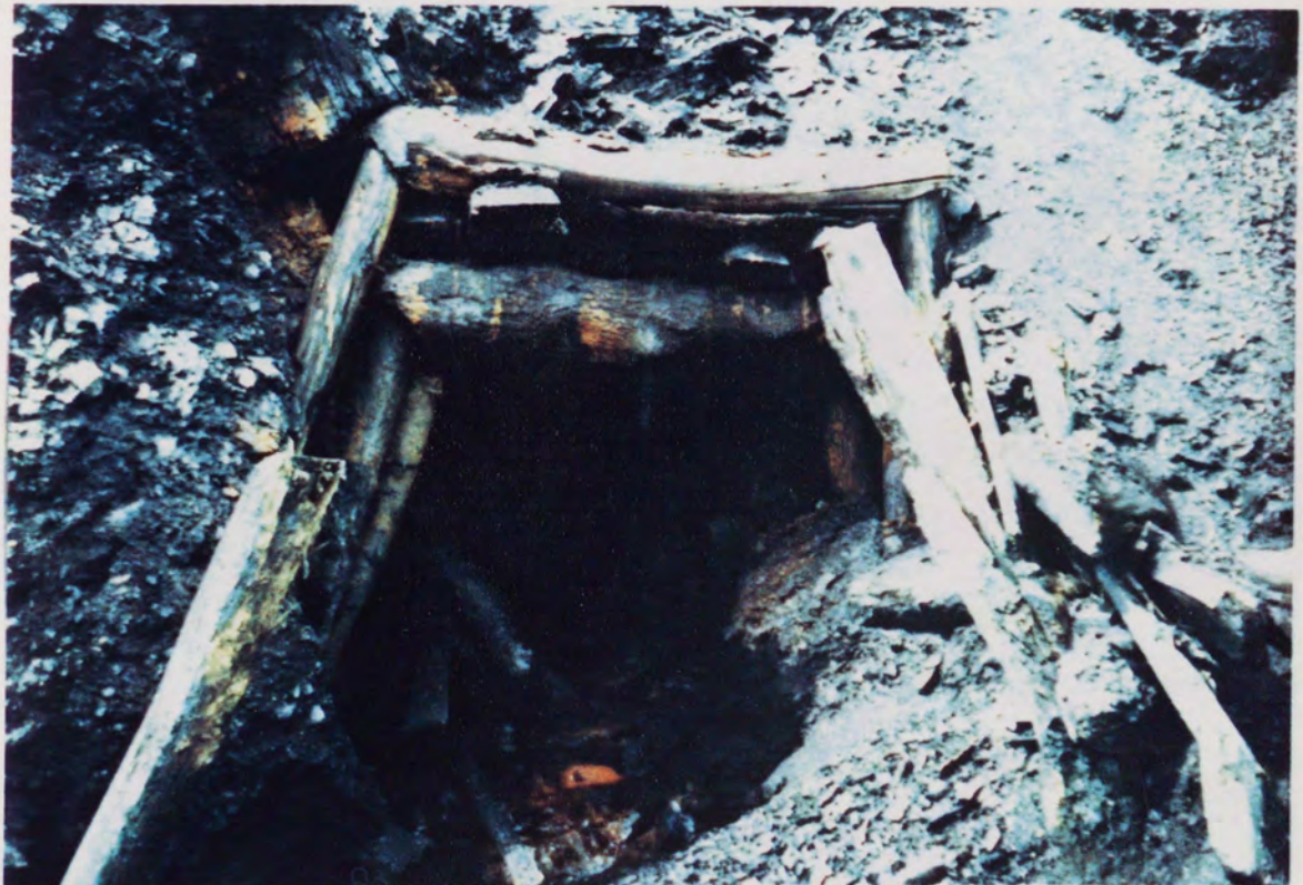
PLATE 5-3-10 Open gallery in Thick coal - north end of western highwall March, 1985.
