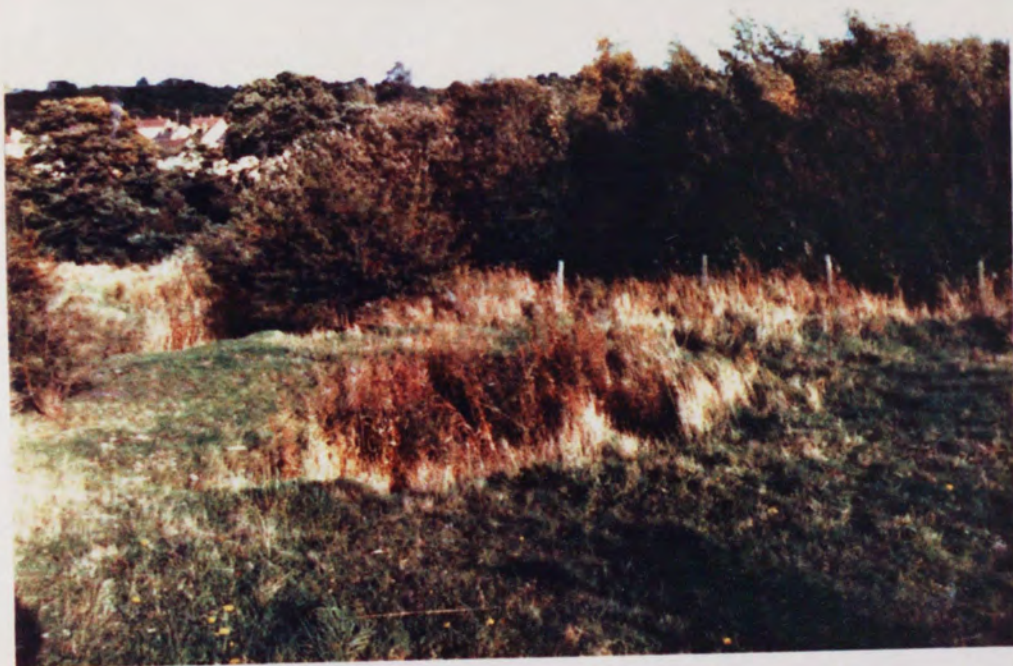
PLATE 5-3-1 'Crown holes' close to south east corner of site. Oct, 1983.
