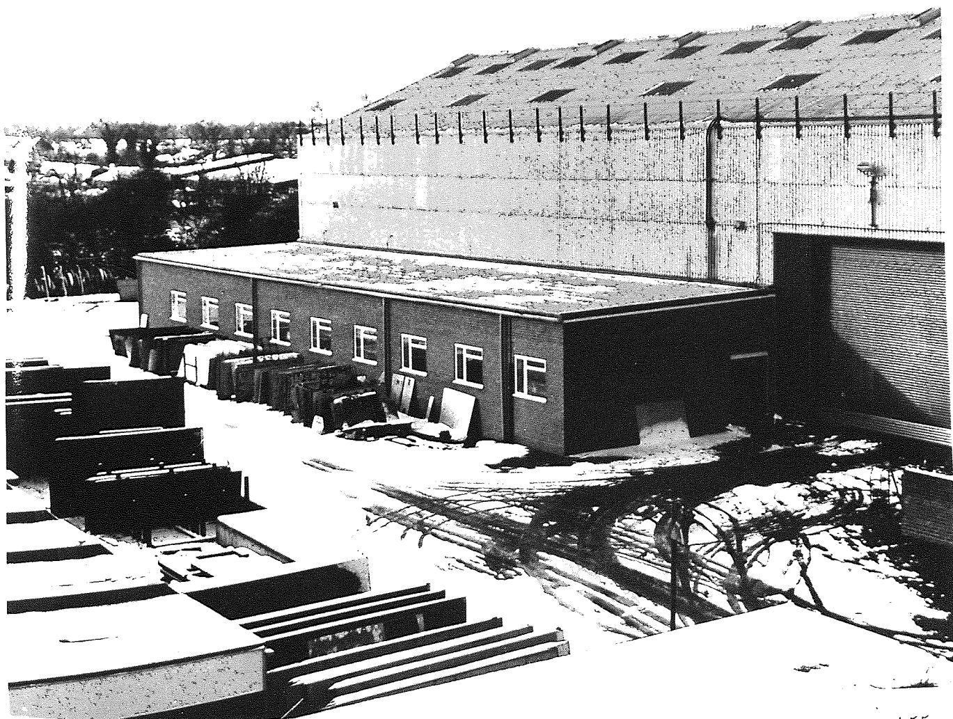
Figures 3.13 and 3.14 Block 55 Annexe - Heat Bridge effect (time interval between photographs 30 minutes)
