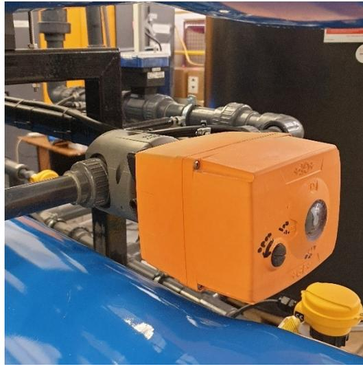
**Fig. 3.11.** Brine flow control modulation valve.
