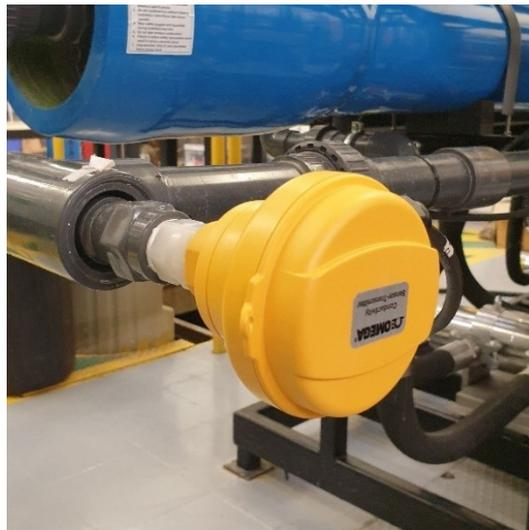
**Fig. 3.14.** Conductivity transmitter.
