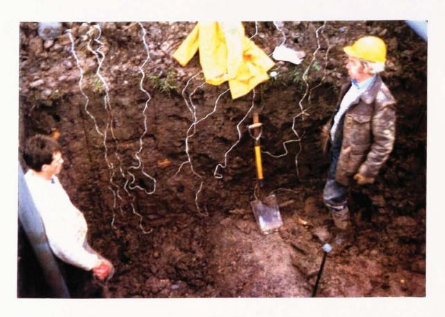
PLATE 7.3 Installation of PRT's at Site C.
