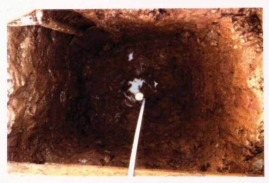
PLATE 7.5 Installation of Soil Pressure Transducers at Site A.
