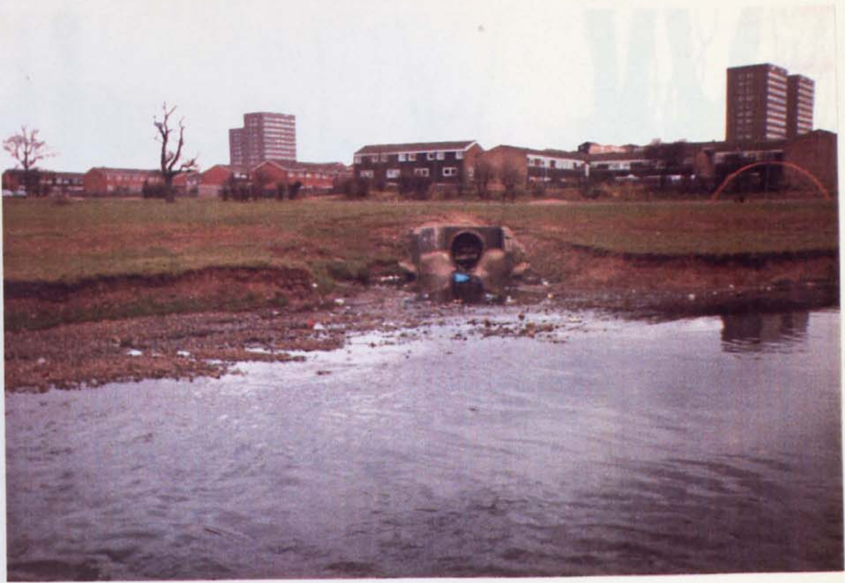
(xi) Site 18 Outfall to R. Cole, Birmingham, with Chelmsley Wood estate in the background
