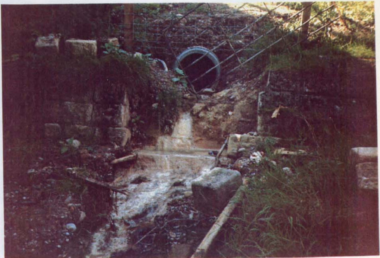
(xii) Site 2 Outfall from construction site to R. Blythe, Solihull
