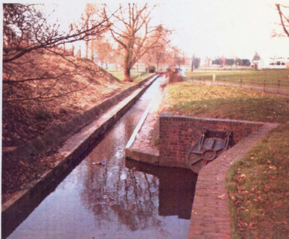
(ii) Outfall to artificial channel, Bromsgrove
