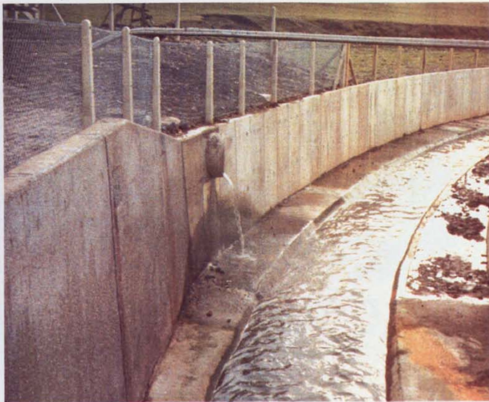
(i) Outfall to artificial channel, Walsall
