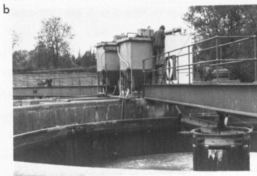
Plate 3.2 LANGLEY MILL PILOT PLANT
