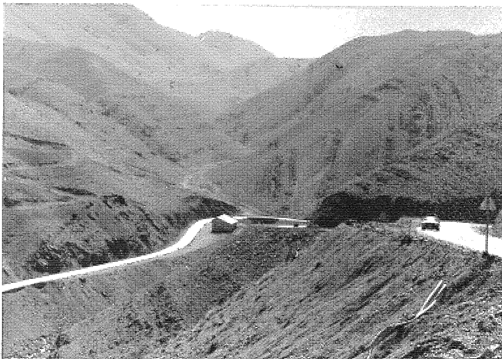
Plate 1.2 Margh valley (km 25). The building is a shelter for passengers who trapped in snow in winter.
