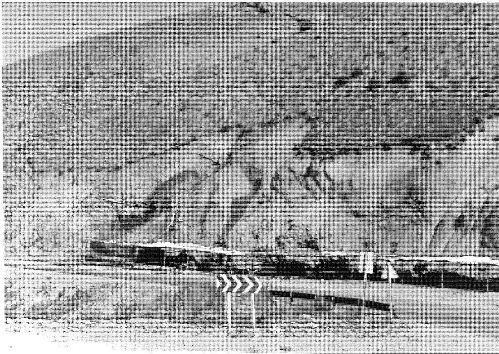
Plate 1.1 North side of the main thrust (km 15). The water flow (→) is consequence of a secondary fault.
