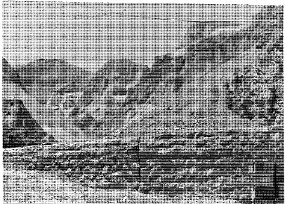
Plate 3.4 Pyroclastics (km 59). The layers are horizontal and they are not affected by tectonic activities.
