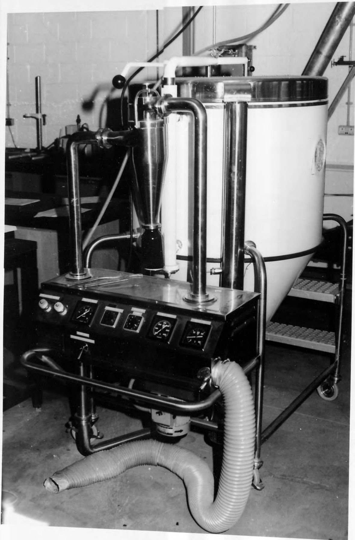
Plate 4.2 Co-Current Spray Drier
